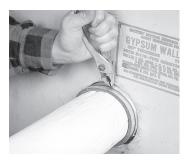
This patented intumescent wrap/strip has 3M state-of-the-art through-penetration fire protection plus improved characteristics.
