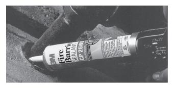
All 3M Fire Barrier Sealants have either intumescent, endothermic or ablative technologies designed to provide a tight and dependable seal against fire, smoke, toxic fumes and moisture. 3M intumescent sealants expand up to 10 times their original size when exposed to temperatures over 300°F (149°C). This intumescent action forms a strong, insulating char that seals the opening for up to four hours when exposed to extreme heat.
