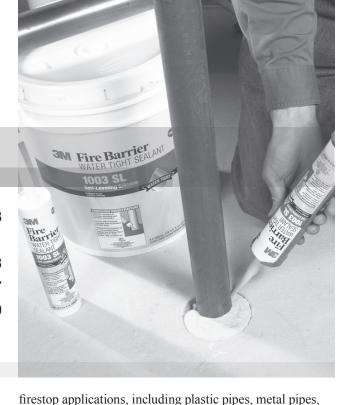
The complete line of 3M fire protection products helps prevent fire, smoke, toxic fumes and moisture from passing through penetrations in fire-rated walls and floors. These easy-to-install products are suitable for a wide variety of
